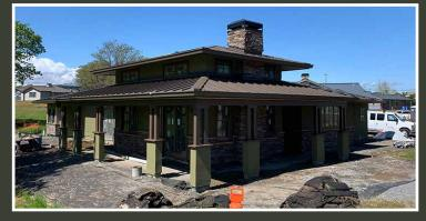
All structures on this project will utilize our standing seam 16" and 18" Design Span® hp metal roofing fabricated out of our 100% renewable and Red List Free ZINCALUME® coated steel. A mix of our energy efficient Cool Dura Tech™ 5000 (PVDF) paint system will be used on the Design Span® hp roof panels which includes a mix of 24ga and 22ga Cool Slate Gray, Cool
