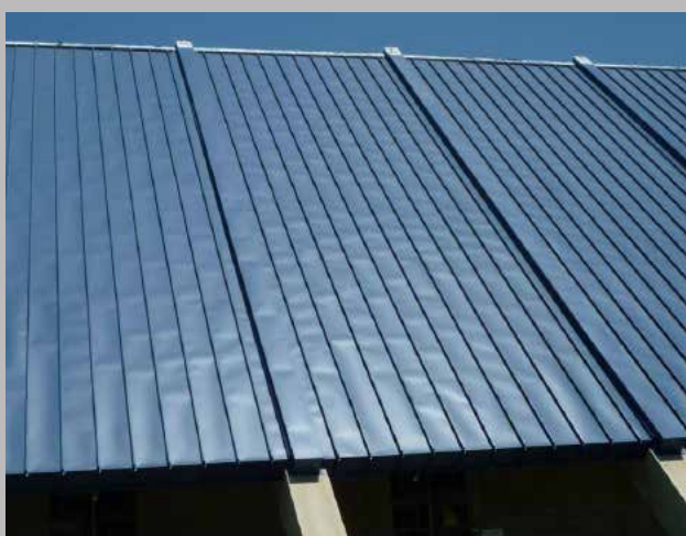
Thermally locked panels fixed at ridge and the roof to wall transition.
