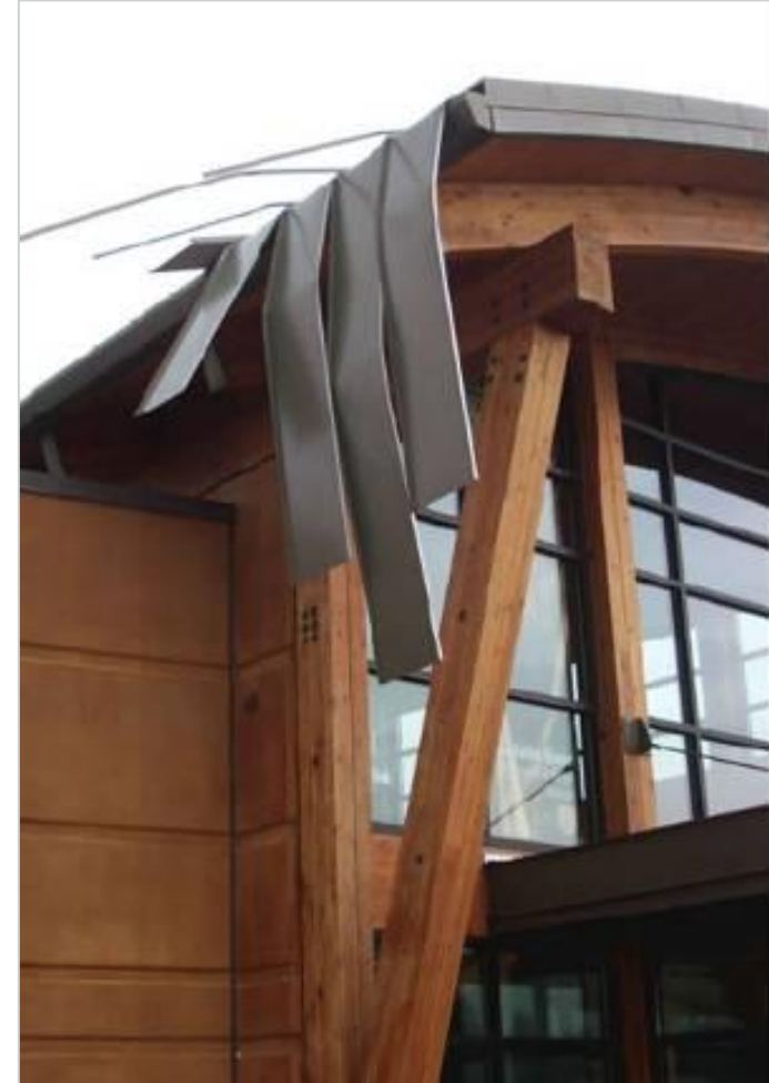
Damaged panels caused by snow drag load.
