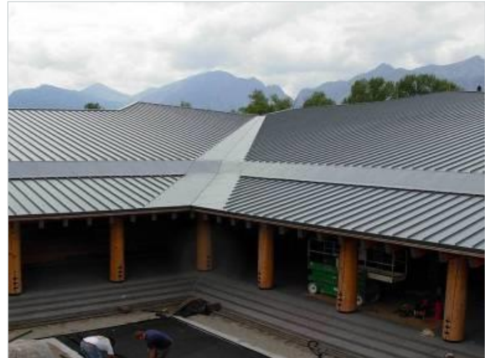
Snow conditions require a special valley design
