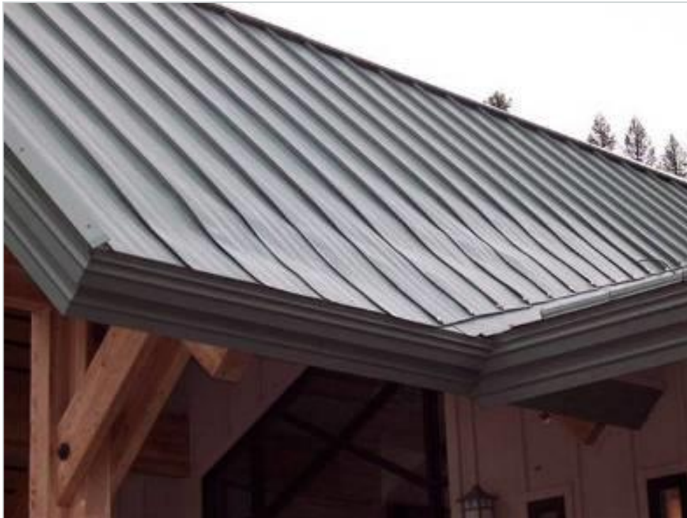
Ribs crushed due to inadequate valley width
