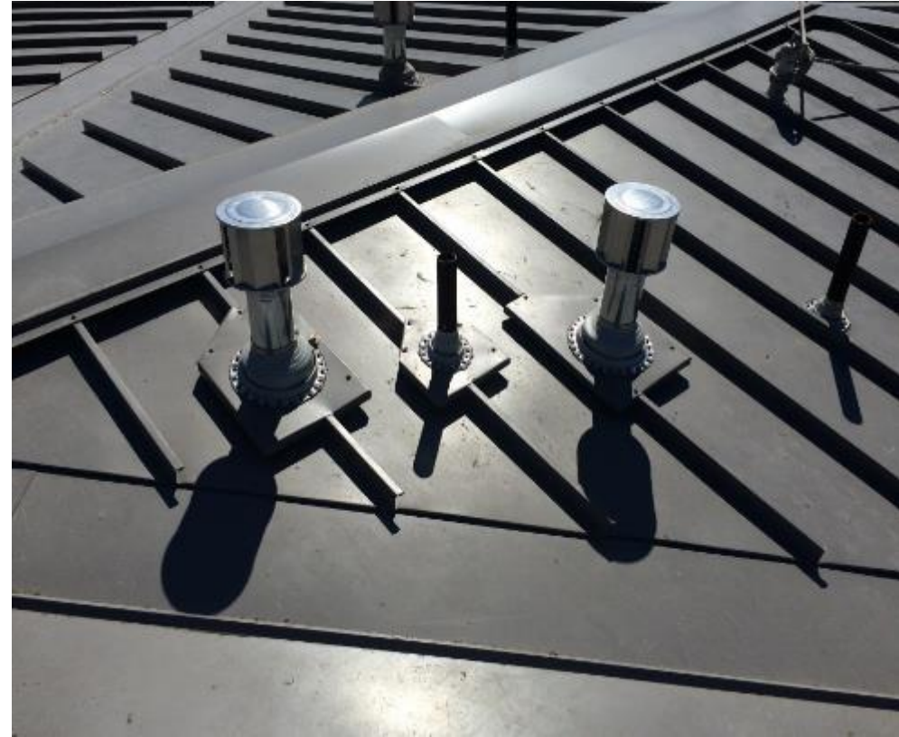
Correct: Cut Rib Detail
