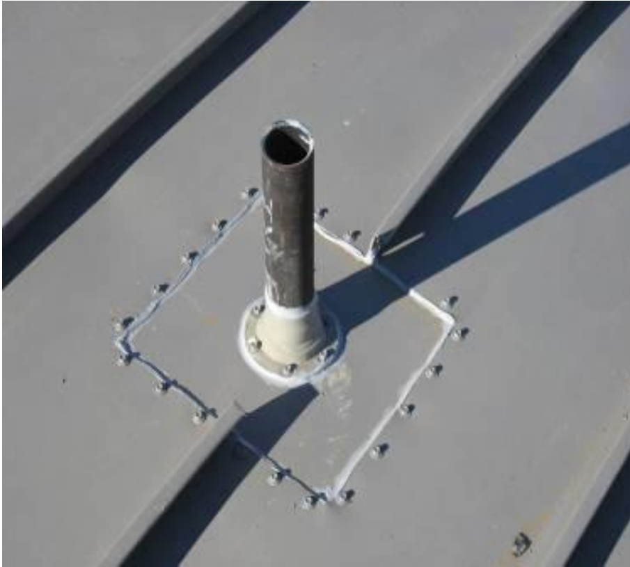
Incorrect: Standing Seam Penetrated
