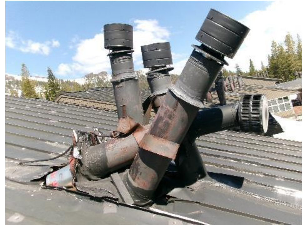
Damage caused by snow & ice build up
