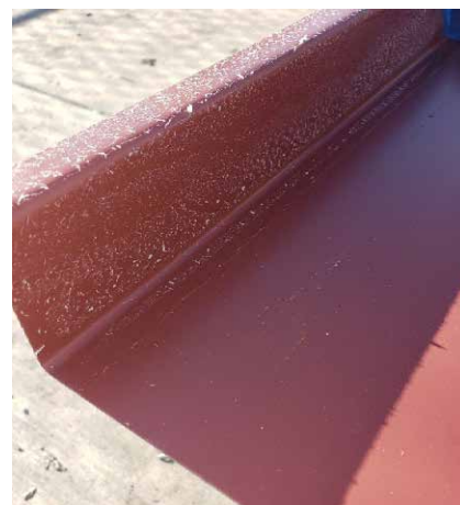
Example of leftover adhesive residue on panel leg.
