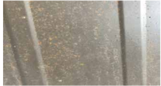
Heavy swarf staining on pre-painted steel.
