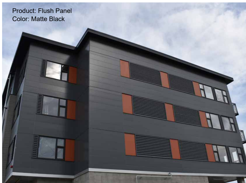
Vented Flush Panel with 2 pencil ribs
