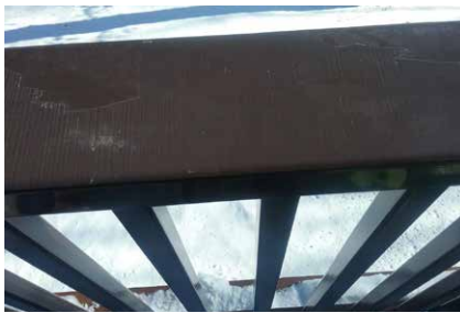
Example of peel coat removed in freezing conditions.
