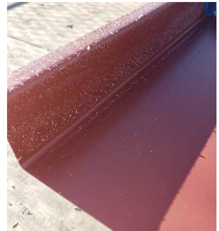
Example of leftover adhesive residue on panel leg.
